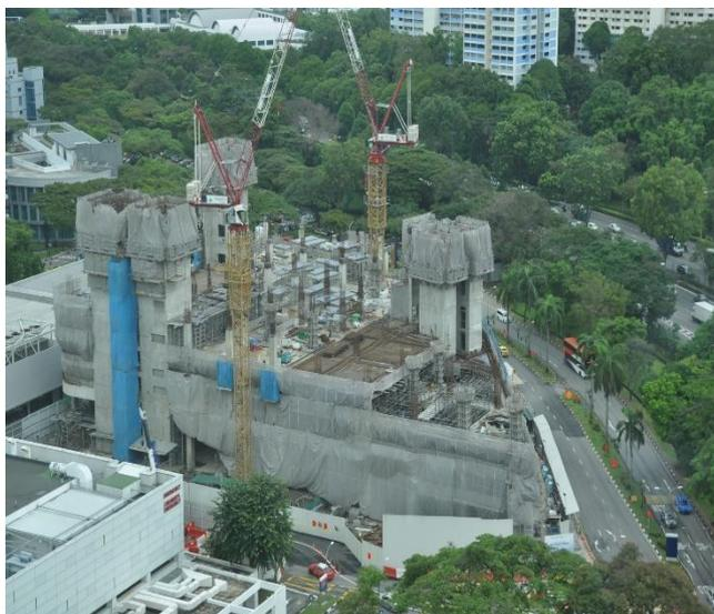
The main contractor for the construction of the National University Centre for Oral Health, Singapore (NUCOHS) commenced work on 1 February 2016. Significant construction activities in 2016 included the completion of piling and excavation works and the erection of the megatruss to cover NUH's existing cooling systems. As you pass by the site today, you would have probably seen a pair of tower cranes, the lift corewalls and the building superstructure from ground level to the 3rd storey.
